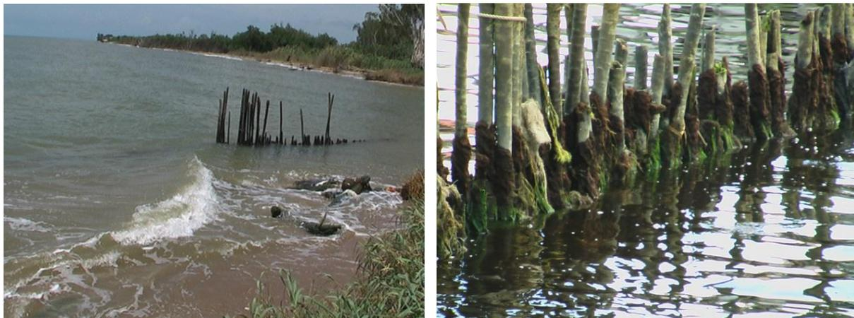
Figure 8.2.2 Palmetto fence ineffective in catalyzing accretion on this sediment starved coastline
