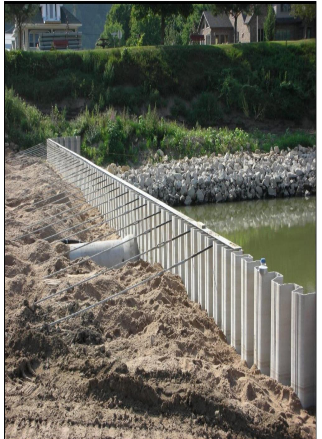
Figure 10.2.4 Examples of vinyl sheet pile walls under construction
