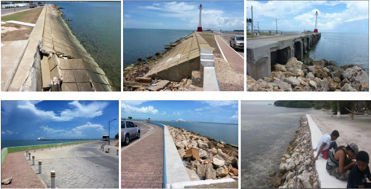
Figure 8.1.1. Examples of seawalls constructed on segments of the Belize coastline
